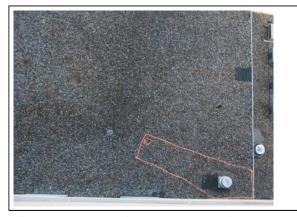
View from above of wet area in expanded polystyrene insulation. Outside temperature +/- 73°F.
